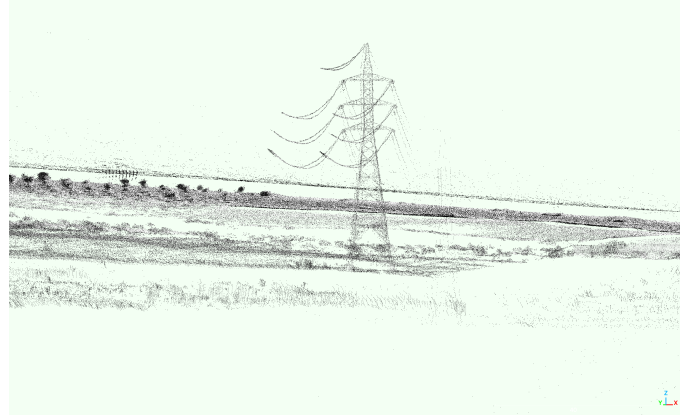
Fig. 5. LiDAR reconstruction of a power transmission tower
